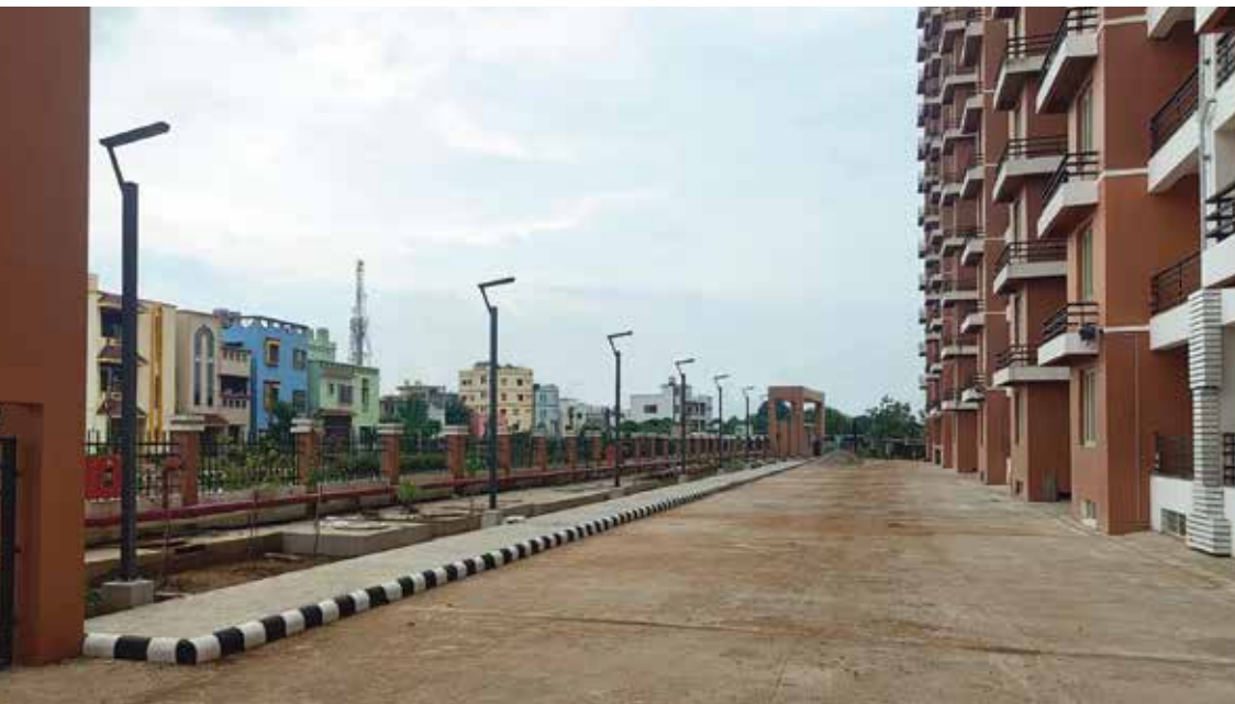
BDA HOUSING PROJECT-SUBUDHIPUR, BHUBANESWAR
